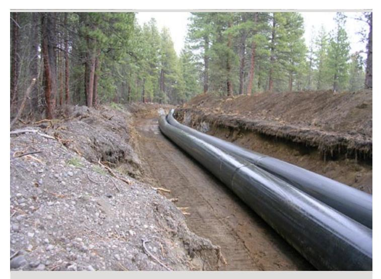
The Deschutes River Conservancy's water conservation project with the Three Sisters Irrigation District piped 3.8 mile section of their main canal located near Whychus Creek in Sisters, Oregon. Piping this section reduces water loss from leaking canal beds and enables the irrigation district to leave 6 cfs (3.8 million gallons of water per day) instream during the irrigation season. Photo courtesy of the Deschutes River Conservancy.
