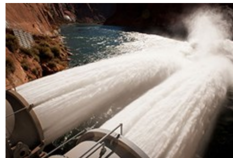
Water being released from Glen Canyon Dam river outlet tubes during 2013 High Flow Experiment
